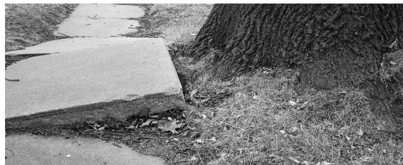
Add a small concrete or asphalt "ramp" to reduce tripping.
