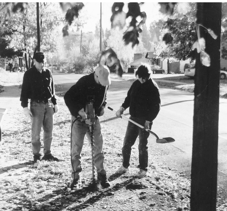
Arborists work not only in trees but in the ground beneath trees. Here a professional arborist volunteers his time to work with tree board members in his community. The group is drilling holes with a soil auger in an attempt to save street trees suffering from heavily compacted soil.
