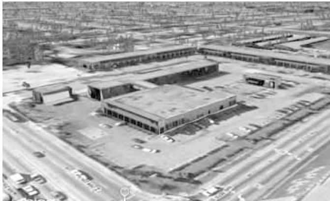
An example of existing distressed property
