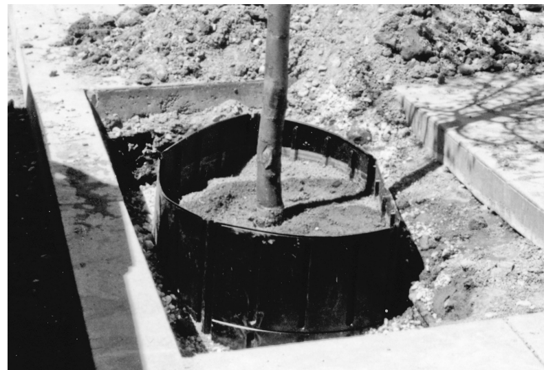
Whether using a solid material or fabric available on the market, a barrier can help direct roots away from beneath sidewalks.
