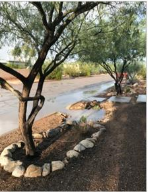
Roots of tree planted next to a curb cut basin grow to access soil moisture under the basin
